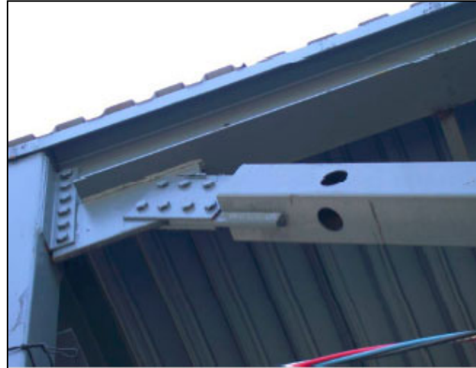
Fusible - contreventement Source: Tremblay, 2011
