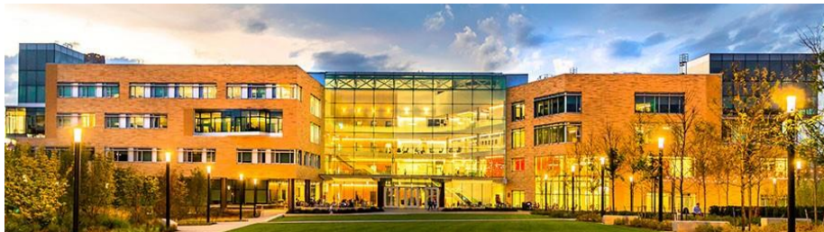
Figure 1 – Le nouveau bâtiment de la Tepper School of Business.
